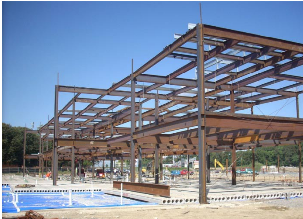
Figure 2: Precast Floor Planks
